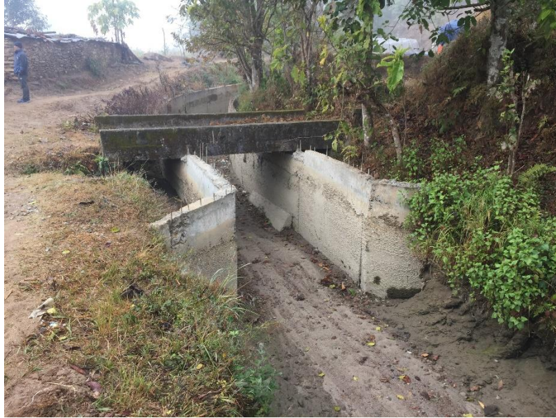
Photograph 9: Rainas Irrigation Canal
