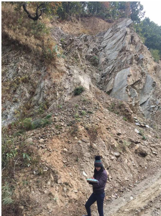
Photograph 2: Study of landslide in the river corridor
