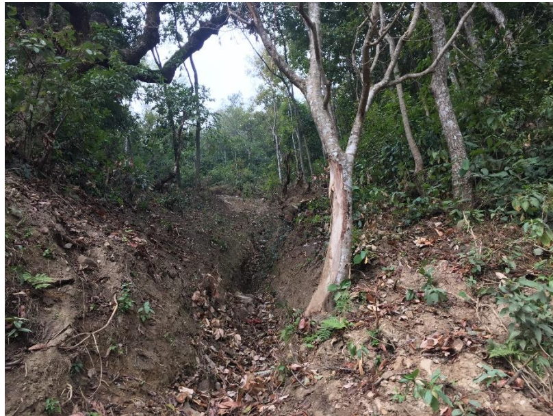
Photograph 8: Created gully resulting the landslide (Rainas, Lamjung)
